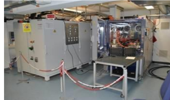
Environment test rig for power electronic units
